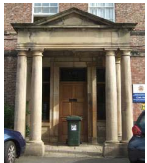
High quality doorways give buildings status, the Hall
