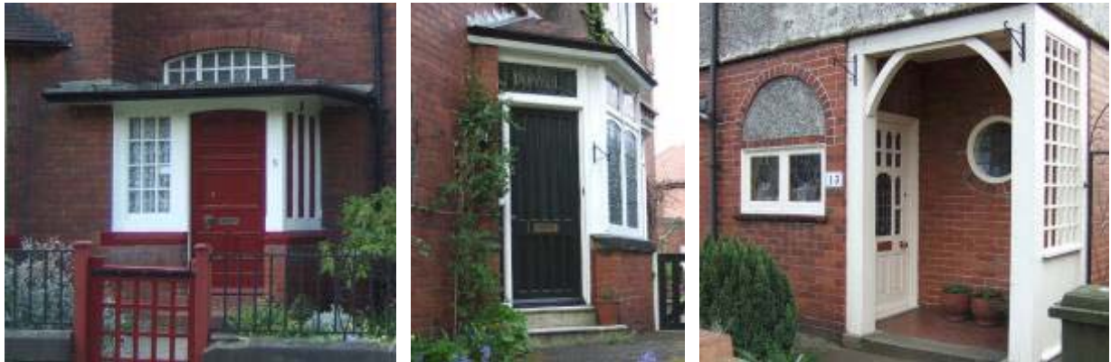
Above, below, bottom: variety of late Victorian, Edwardian and 1920s/1930s doorways ((Park villas, Kings Road South, Grange Villas)
