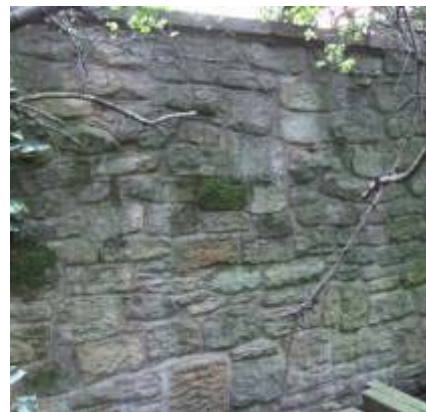
Rebuilt local sandstone boundary wall, The Villa
