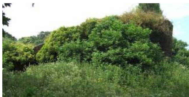
Overgrown Vinery walls, Hall Grounds
