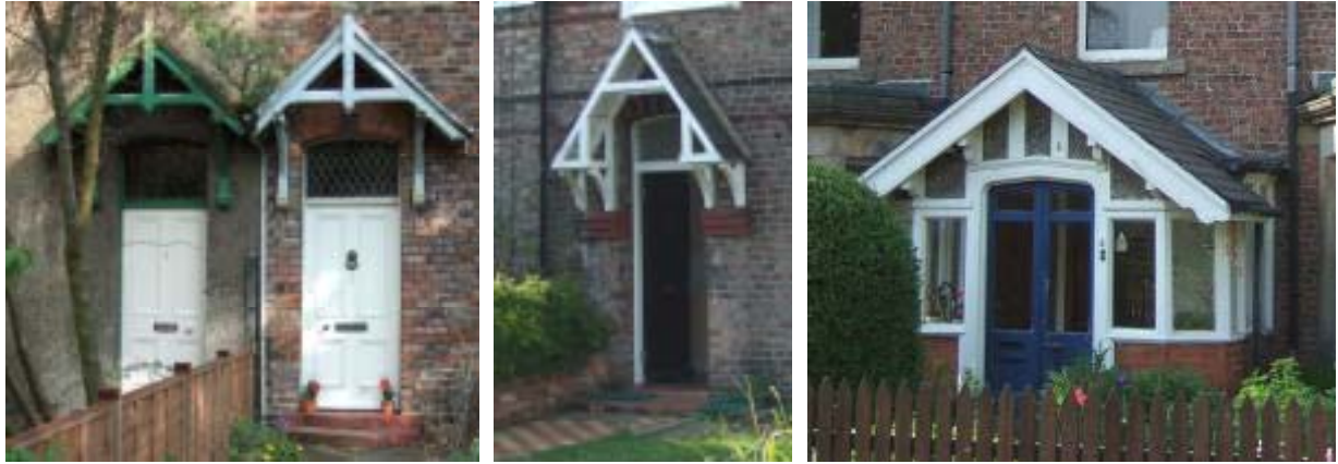
Above: Victorian doorways with timber hoods on brackets, and an ornate half-glazed porch (East and West Vilas, Elm Terrace)
