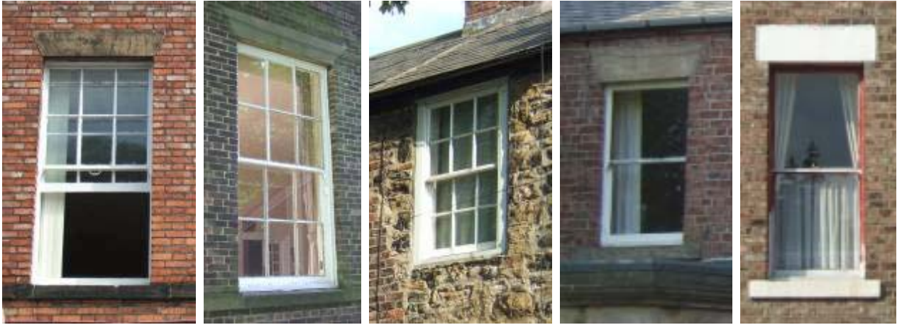
Victorian and reproduction Victorian sliding sash windows, some with glazing bars, some with horns, some with both
