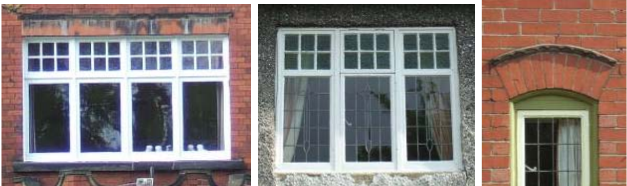
Edwardian & 1920s/1930s timber casement windows, vertically proportioned, with beading and coloured/textured glass in the top light. Below: painted leaded glass. Right: traditional 1920s/1930s colour scheme
