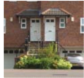
South Sub-Area doorways emphasised with hoods
