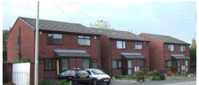
Chimneys are well used in some recent housing (eg. Whitehouse Mews, left) but the roofscape is deadened where they are omitted (Morgan Vs, above)
