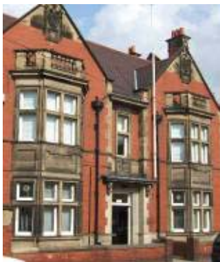
Well weathered sandstone detailing should remain unpainted
