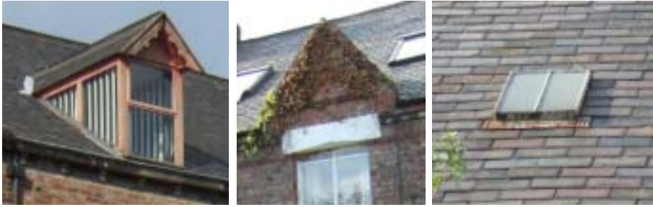
Traditional Victorian dormer, Dene Hse; peaks above 1st floor windows & early metal rooflights, Elm Tce
