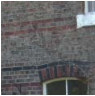
Polychromatic brickwork, Elm Terrace and West villa
