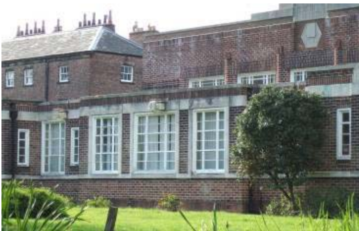
Characteristic Art Deco timber and metal windows, Health Centre
