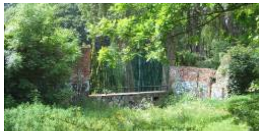
Important but ruinous vinery walls and other structures
