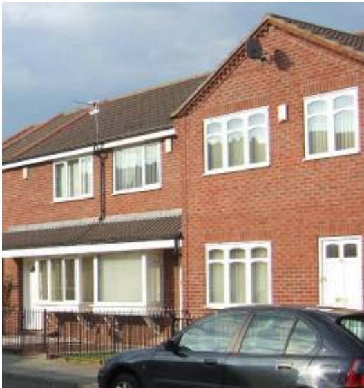
Windows in the South Sub-Area
