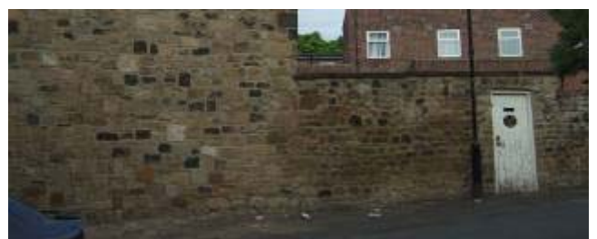
Secluded back gardens and historic garden boundary walls, some rebuilt
