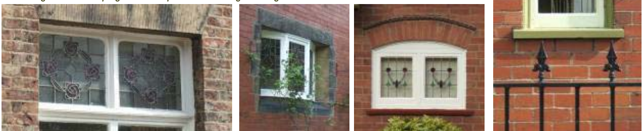
Edwardian & 1920s/1930s timber casement windows, vertically proportioned, with beading and coloured/textured glass in the top light. Below: painted leaded glass. Right: traditional 1920s/1930s colour scheme
