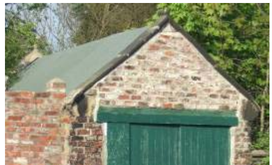
Verges have stone water-tabling, those on Boyd St's outbuildings with high status roll-topped ridge blocks and moulded kneelers
