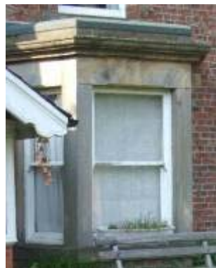
Well weathered sandstone detailing should remain unpainted
