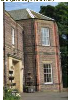
Interesting forms: side pavilions (Whitehouse Mews) and robust angled bays (the Hall)
